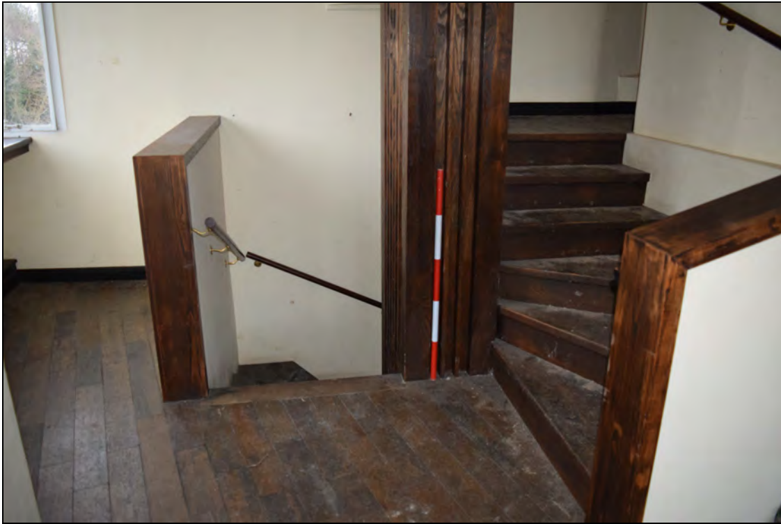
Figure 27: The top of the stairs connecting the ground floor and basement at the northwest corner of the mid-Victorian wing of the hotel, which will be replaced (B2). It is thought to be non-original, and its surroundings appear modern, but its fabric should be checked during removal to ensure the modern fabric does not obscure an earlier arrangement.
