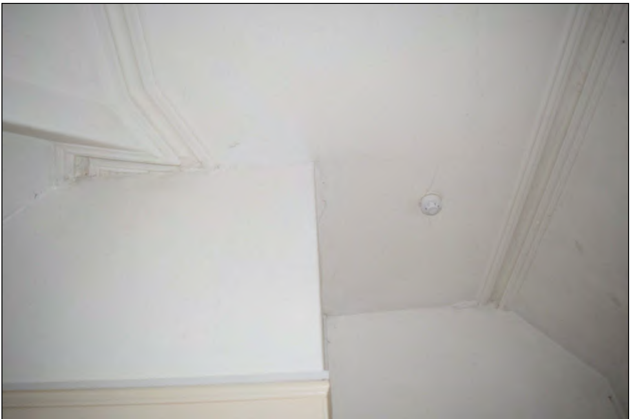
Figure 33: The ceilings of the first-floor rooms at the northwestern corner of the hotel at first floor level show that the mid-Victorian rooms have been subdivided by later stud walling, with original plaster coving cut by the later walls. Removing some of these later walls (FF1) may restore some rooms to a condition closer to their original form. The date of the stud walling is not always clear, however, and could range from late-Victorian to late 20 th century, hence this work needs to be monitored and recorded where historic fabric is revealed or removed.
