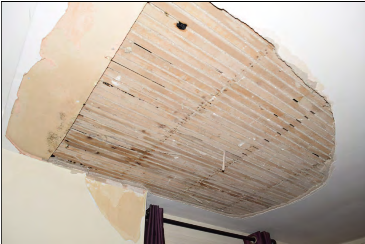
Figure 37: A damaged section of ceiling on the second floor of the Victorian wing of the hotel facing Bridge Street reveals original laths beneath the plasterwork.
