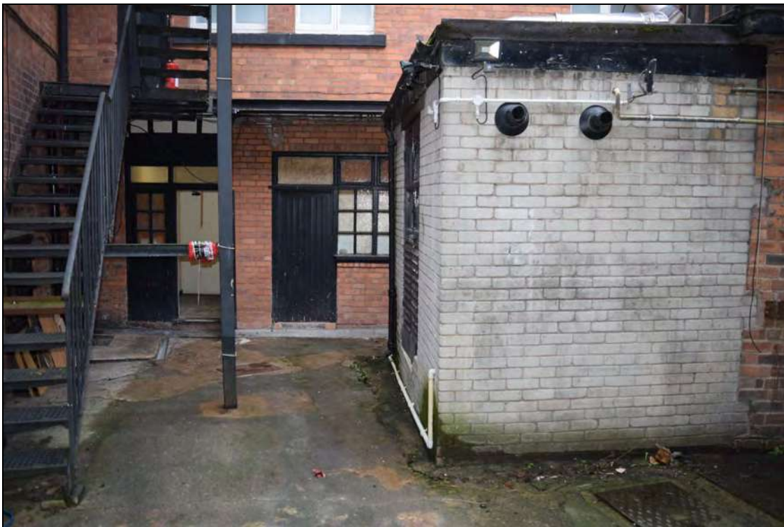
Figure 28: (right above): The central courtyard is at basement level. The brickwork is late 19 th century in date and appears to have been built between the publication of the 1880 and 1900 1:10560 Ordnance Survey maps. There are also 20 th century elements, such as the block seen to the right of centre, which do not appear on the 1900 Ordnance Survey map. The facing doors will be widened (B5 & B6) and their fabric should be recorded before removal.
