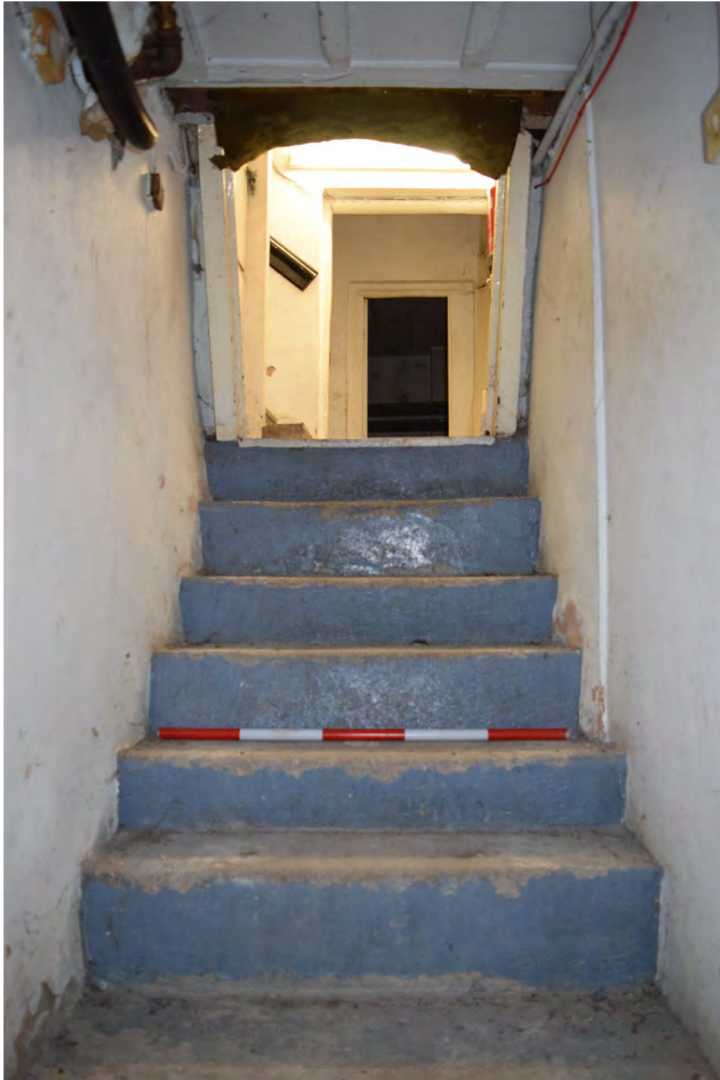
Figure 29: The steps leading from basement level down to the sub-basement level, which lies beneath the Georgian "New Hotel", B24. The date of this access point is not known but the steps appear to be relatively modern concrete. Work to modify this access point to the sub-basement to increase headroom may reveal original fabric and should be monitored.
